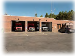
9 th Street, Station 2 410 9 th Street
