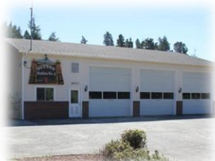
Sutton, Station 4 88973 Sutton Lake Rd
