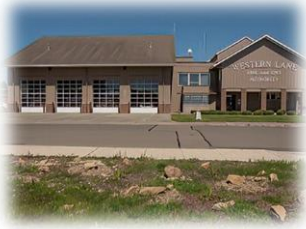
Central, Station 1 2625 Highway 101
