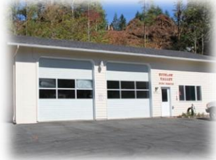
North Fork, Station 6 9181 North Fork Rd
