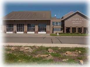
Central, Station 1 2625 Highway 101
