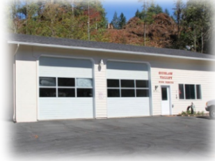
North Fork, Station 6 9181 North Fork Rd
